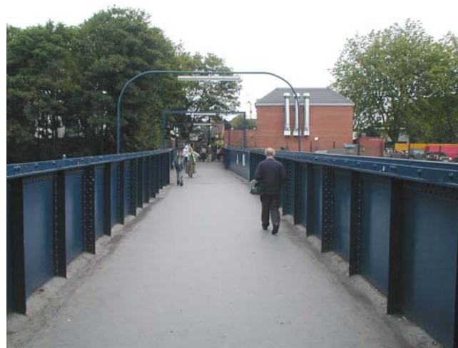
Footbridge between High Town and town centre is functional but lacks character and amenity
