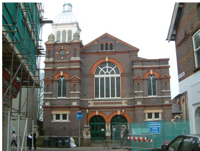
The Methodist Church is both a key landmark and a key community facility
